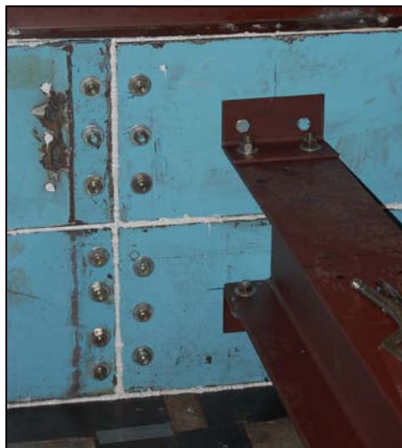
Figure 3.8. Purlin Support Beam to Chamber Connection
