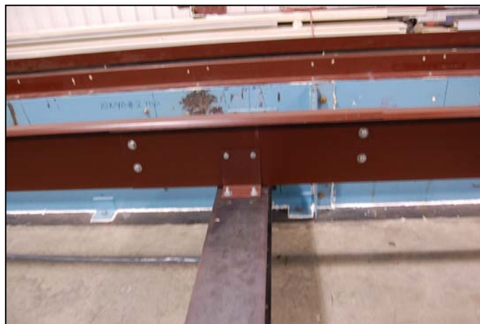
Figure 3.10. Continuous Span Typical Lap Connection
